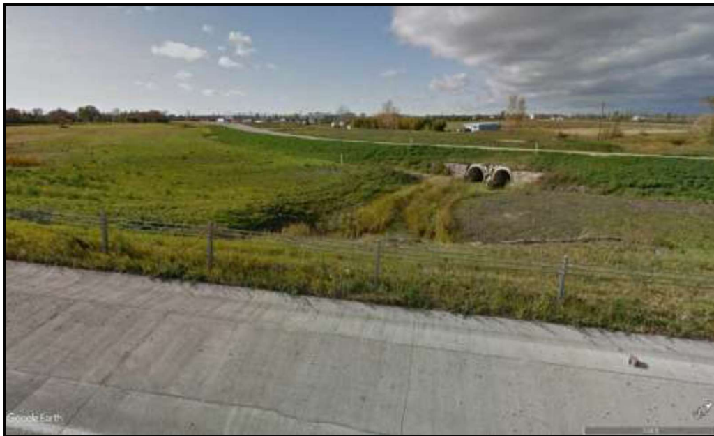
Photo 5. New High-Flow Culverts under Inkster Blvd. to Enhance Capacity.
